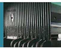
Boiler tubes district heating station can withstand temperature cycling, corrosive environments and fluctuating particulate levels.
